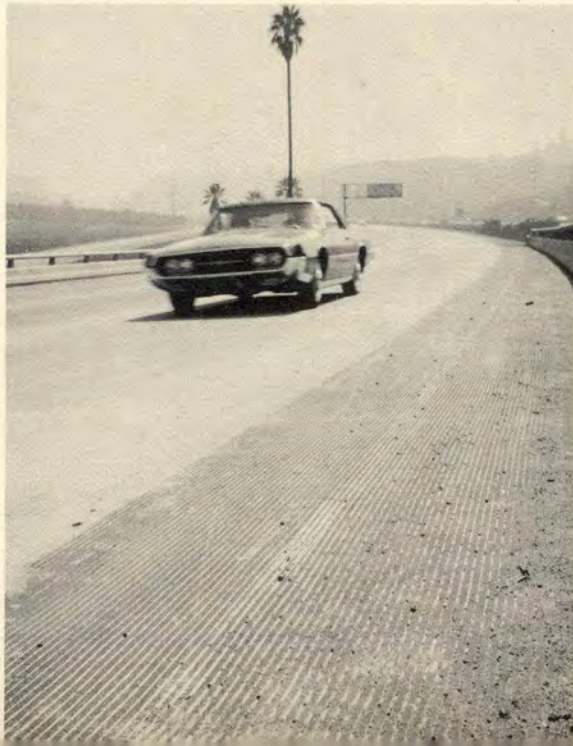
Grooved pavement on California freeway. Grooves run parallel to roadway, whereas runway grooves are transverse for best effect.
