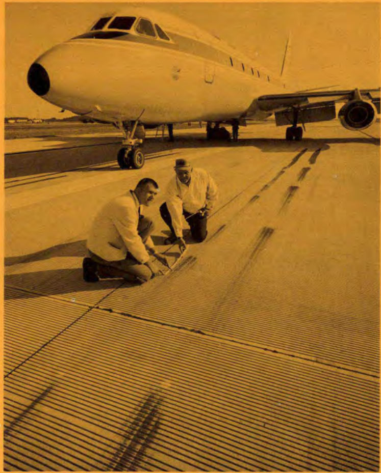
Mr Walter Horne and Mr Thomas Yager, of the NASA Langley Test Facility, study the touchdown point of Con-vaire 990 in recently completed test on grooved runway at Wallops Island.
